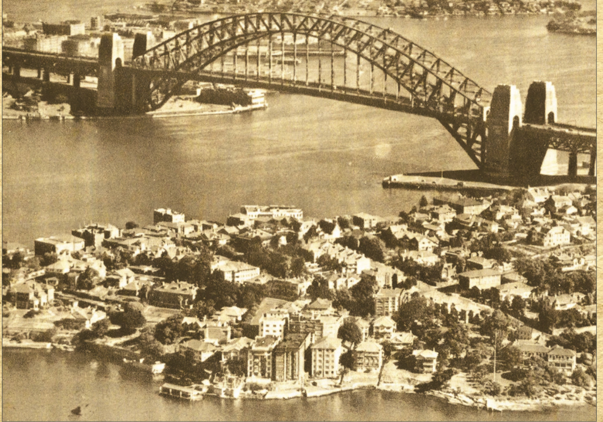
Sydney Harbour Bridge
